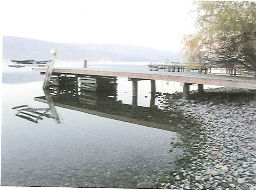
Photograph 8: View of existing dock from the north. Note the two large cribs and concrete pilings and boatlift
