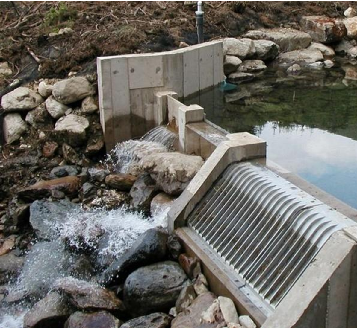
Point #22 Proposed intake with Coanda screen will be built similar to this one.
