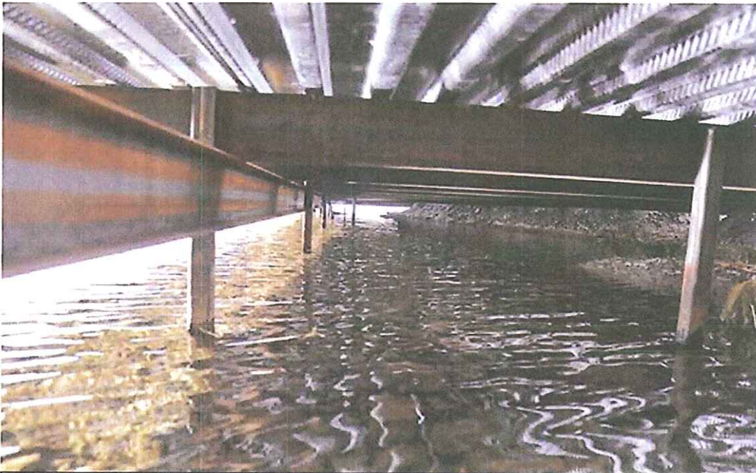
Photo E. View looking west from under the dock structure. There are no rooted aquatic plants under or near this dock that will be shaded by this structure. However a light-penetrating deck material would decrease the amount of shading to phytoplankton.
