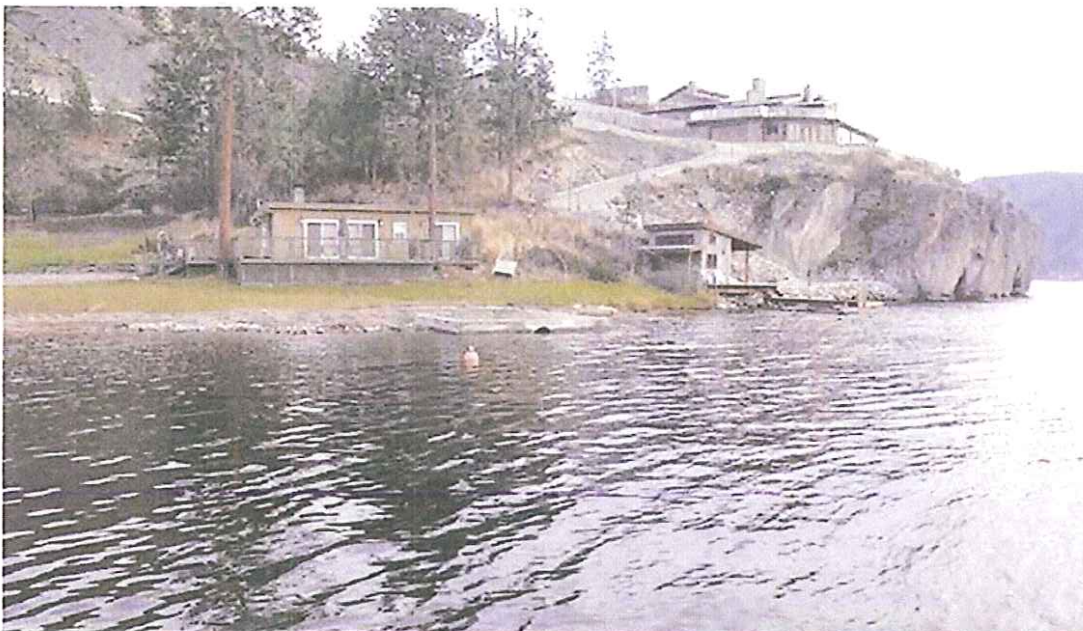
Photo F. View looking south west from the north property boundary along the dock. The foreshore area in front of the cabin and the area to the right of the cabin will be vegetated with 90 native species of plants to off-set the footprint of the proposed structure.
