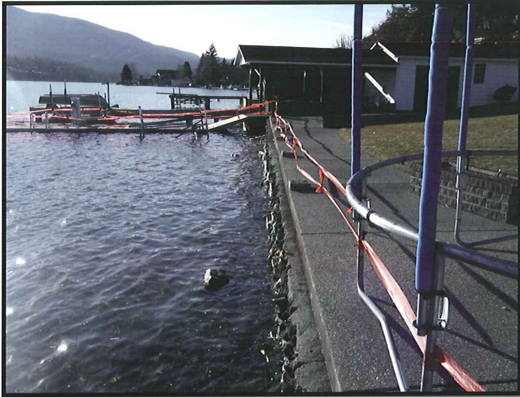
Photo 1 – Foreshore of property looking South
