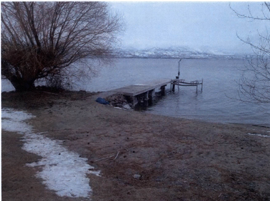
Photo 5) View looking north at the existing dock. This does not conform to the existing provincial guidelines and will be removed. The walkway is greater than 1.5 m and the depth of water at the end of the dock is < 0.8 m at low water. A floating silt curtain will be used when removing the existing pilings as this has the highest potential for sedimentation disturbance.
